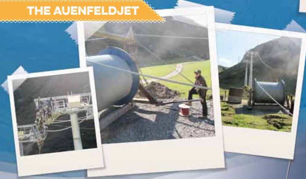
Snapshots of the construction work on the Auenfeldjet: A heavy-lift helicopter hauled the towers - each weighing up to 15 tons - into place.
